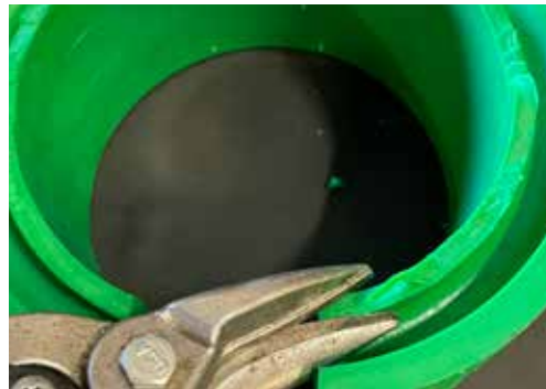
4. Due to the large diameter of the coil, you will need to trim top inner rings to assist in installation.
