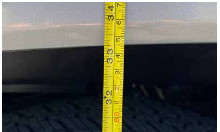
Ground to fence height around 33".
